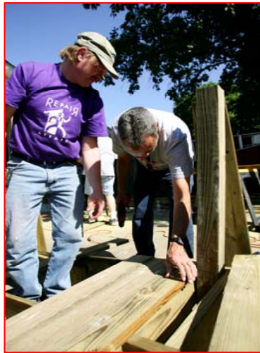
Repair Affair volunteers build a wheelchair ramp.
